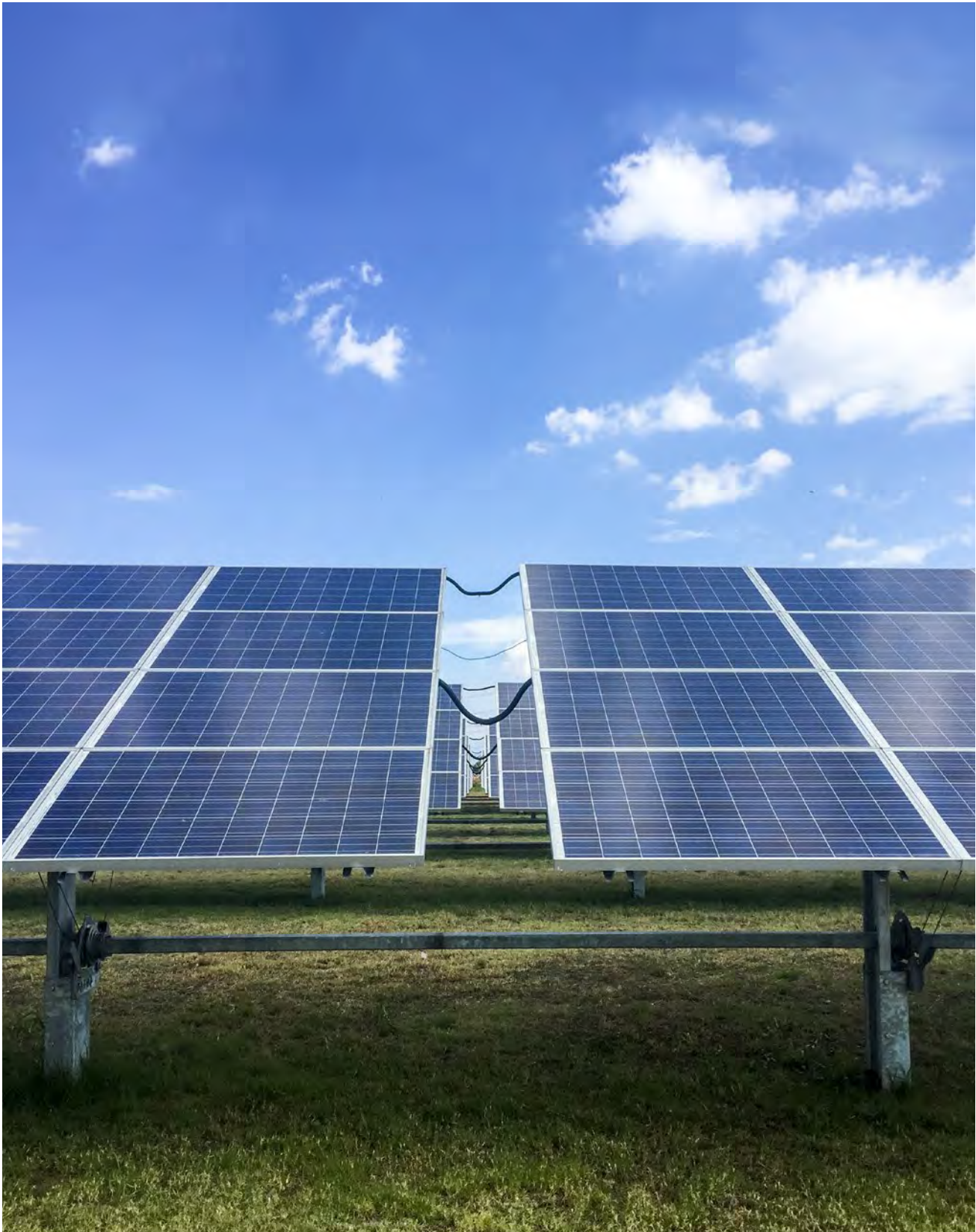
Mexico City, Mexico 20MW
