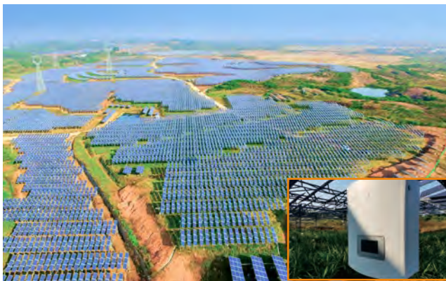
Zhejiang Hangbu Agricultural-photovoltaic hybrid PV plant 30MW
